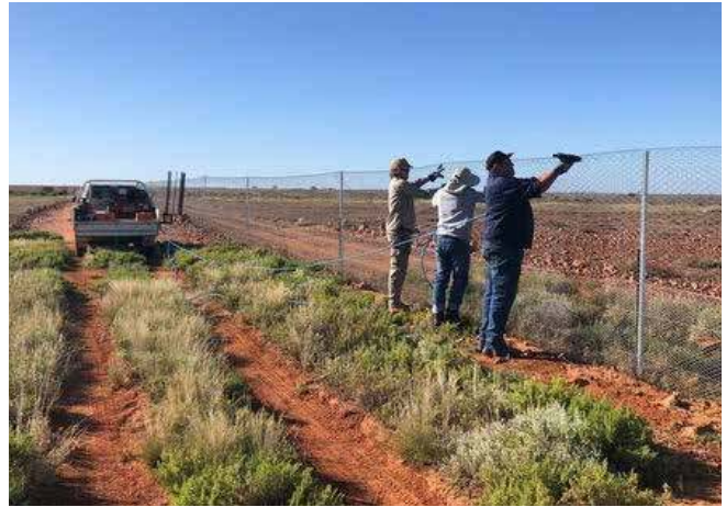
↑ Nathan Manders' team clips new panels of netting to raise the southern boundary of Dingo Pen to 1.8m along the 7km section.
