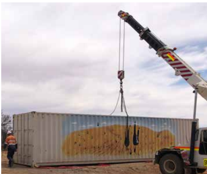
▲ The Ahrens crane repositions a shipping container ready for installation of new solar panels.
