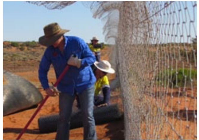
↑ Interim GM Kelli-Jo Kovac and Round 2 Green Army participants replacing footnetting along the western boundary of the Reserve.
